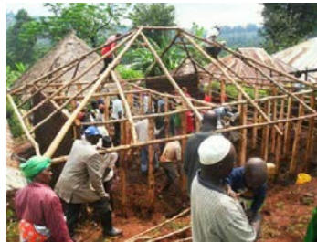
Community members and vol- unteers busy building a house.
